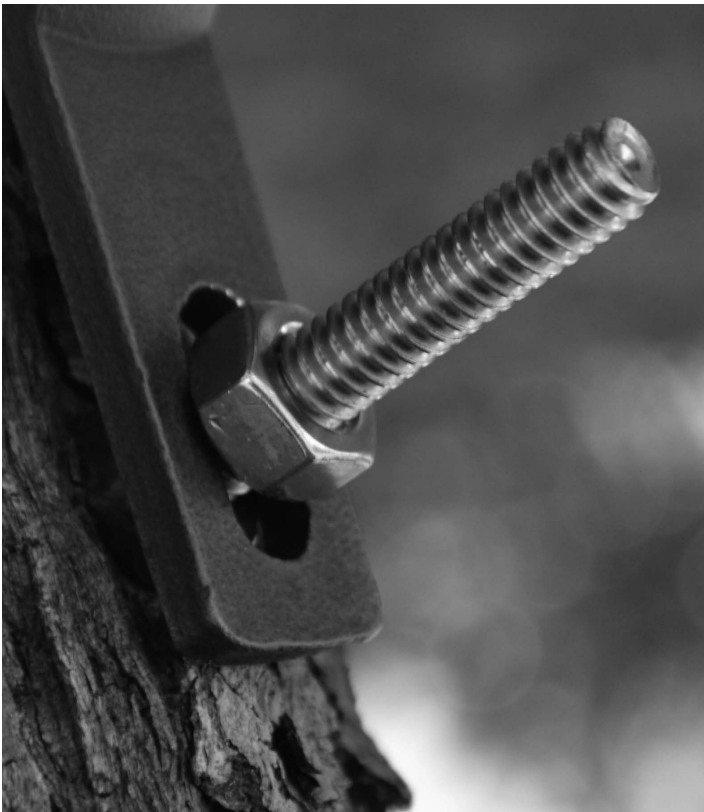
3. Place FA-TB2A bracket over hanger bolts and secure with hex nuts
